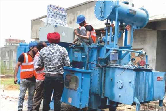
Transformer & BBT Installation
