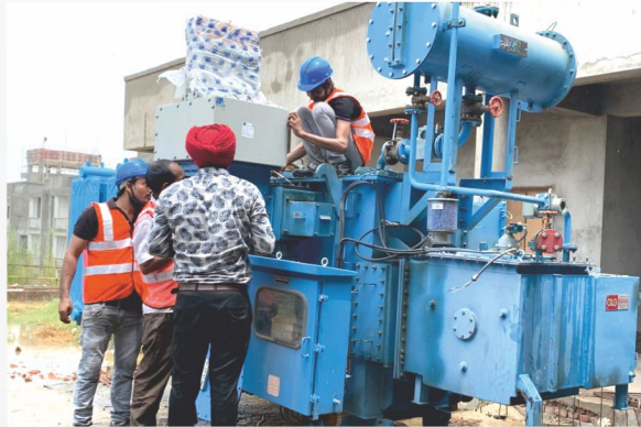
Transformer & BBT Installation
